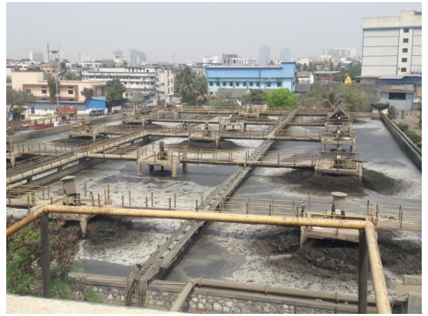
Extended Aeration Tank
